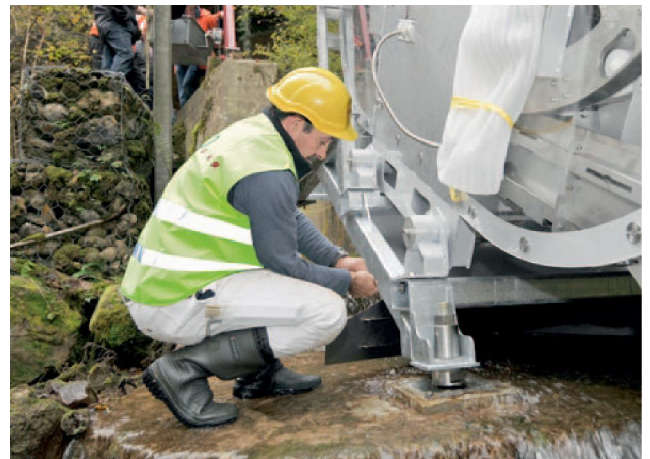
Pilgersteg, Rütli, Switzerland. Installed in three hours. Only four attachment points
