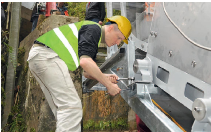
Pilgersteg, Rütli, Switzerland. Installed in three hours. Only four attachment points
