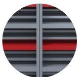
Visible butt joint
