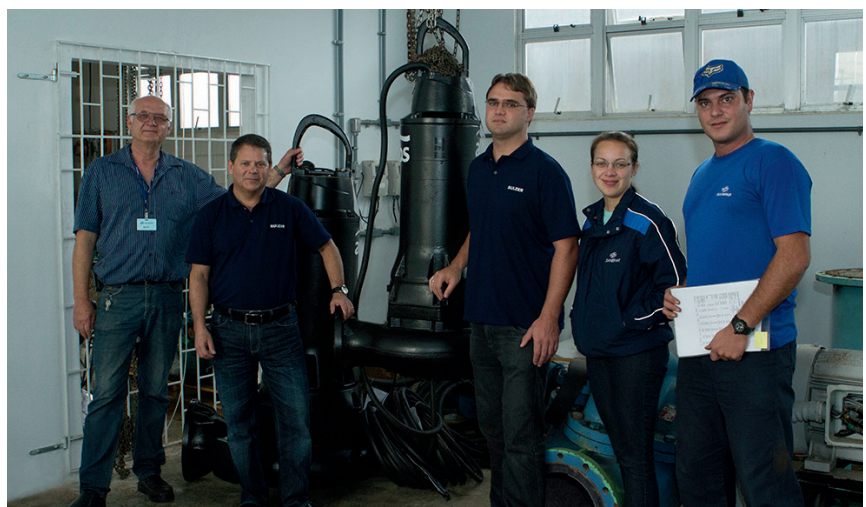
Sanepar staff with an ABS submersible sewage pump XFP
