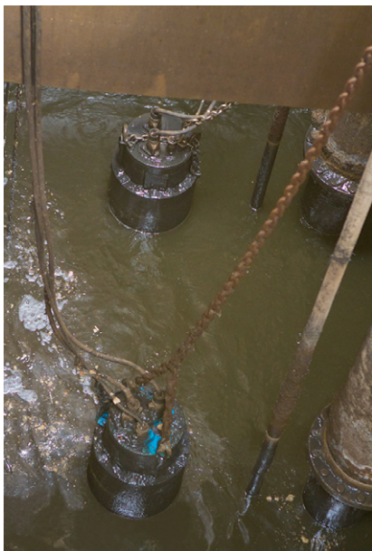
ABS submersible sewage pumps XFP
